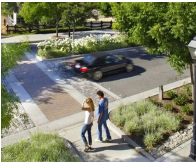
A raised crossing with planted bioretention bumpouts
