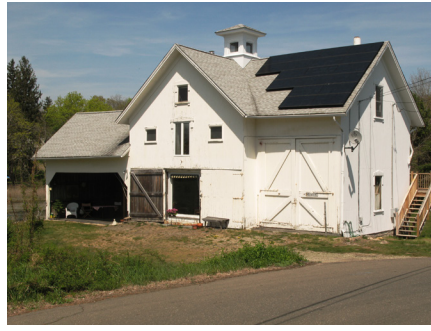
Solar roof panels
